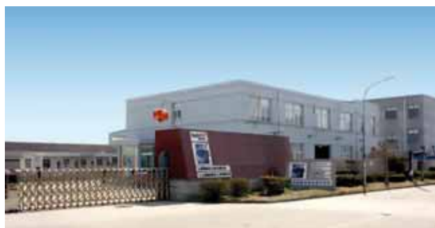
Headquarters - Shanghai - China
